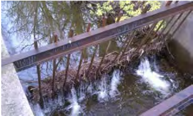
Trash Rack at Gallagher Road End of Mill Race Obstructing Flow
