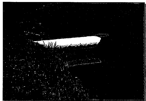
PVC Spillway Pipe
