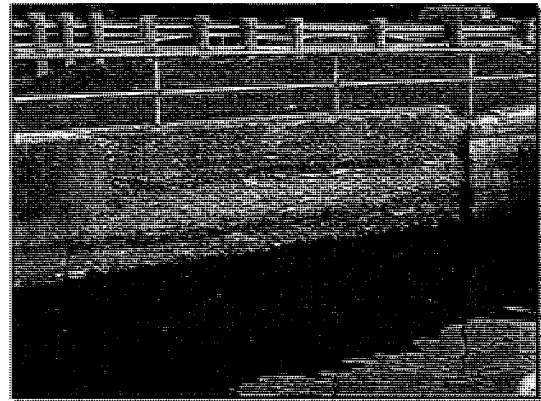
Concrete Spalling
