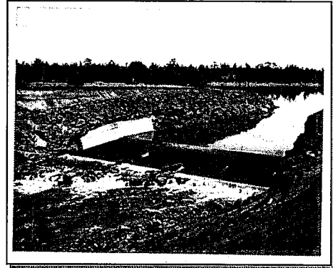
Unlined Earthen Channel Spillway Erosion
