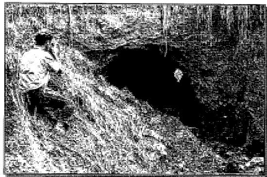
Internal erosion along conduit
