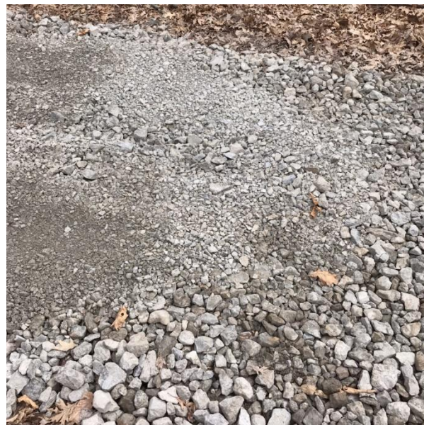
#4, Ditch in previous photo leads to this culvert pipe; note large size gravel for trail base. This is then covered with smaller gravel as shown in the next photo (#5)
