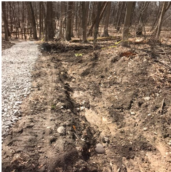
#3, New ditching along very steep trouble spot (camera angle disguises steep slope)
