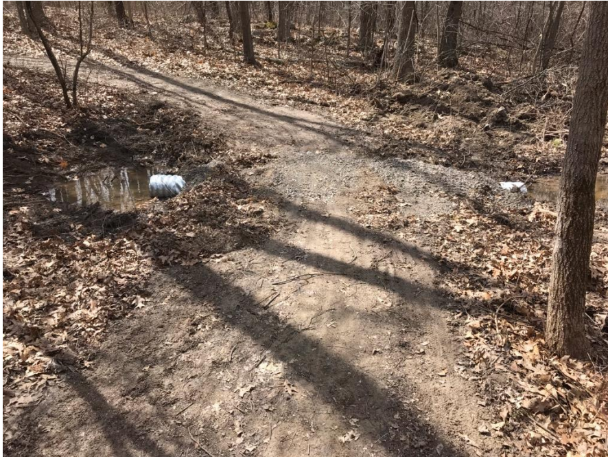
#2, New drainage pipe at often-wet spot near the top
