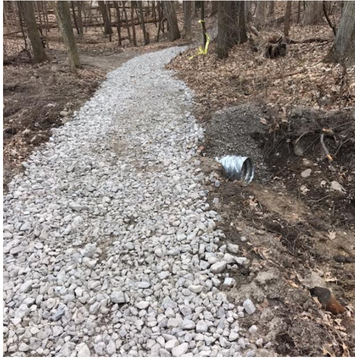
#4, Ditch in previous photo leads to this culvert pipe; note large size gravel for trail base. This is then covered with smaller gravel as shown in the next photo (#5)
